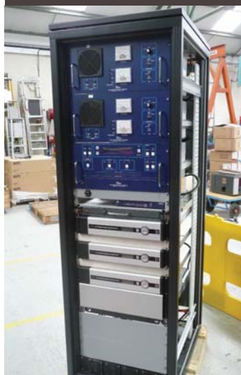
ABOVE: One of the DGPS Racks under Commissioning at VT Systems.
